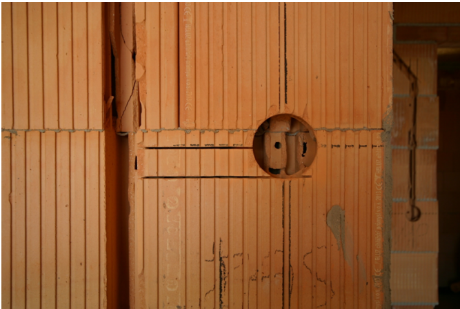
Figure 2: Model slot/switch slot-making and brick cutting using a grinder
