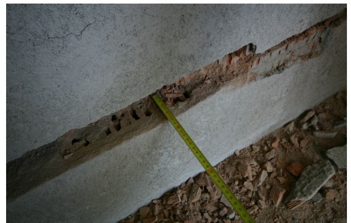
Figure 6: A detail of the electrical box socket area
