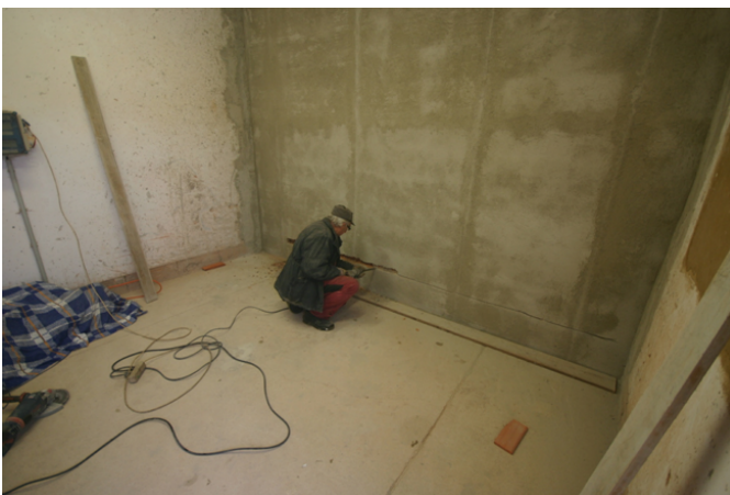
Figure 3: Slot-making – cutting the wall and knocking out the slot
