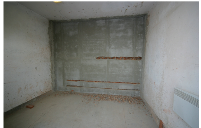
Figure 5: A view of the wall in the source room test laboratory, post-test completion
